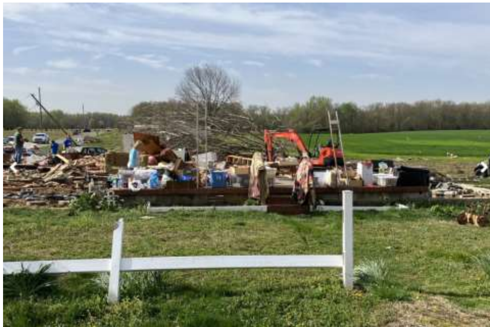
Remnants of a destroyed house on Borderline Rd on the AL/TN border from an EF-3 tornado on April 1, 2023. Photo courtesy of WFAA-48.
